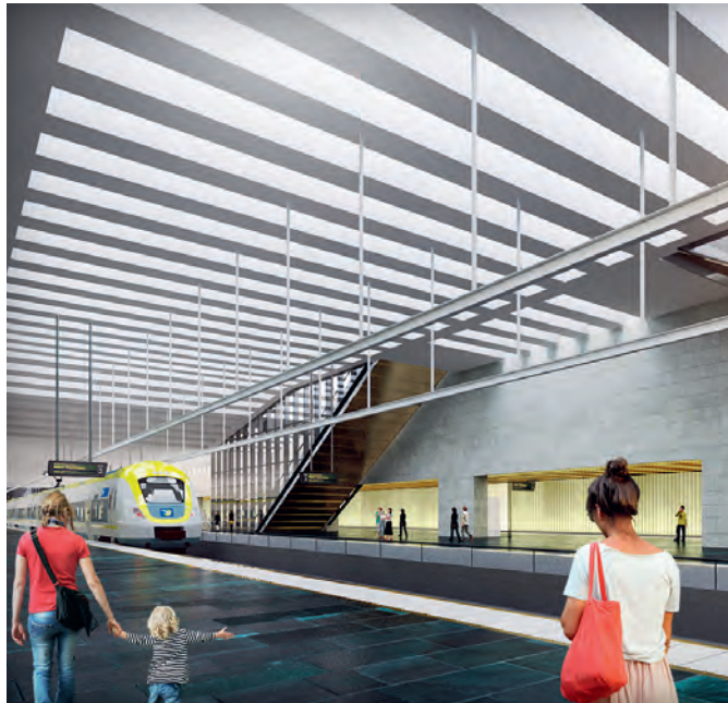
Sketch showing possible future appearance of part of Gothenburg Central Station on the West Link. An important design feature is to allow daylight to penetrate to the interim level. Illustration: White arkitekt.
