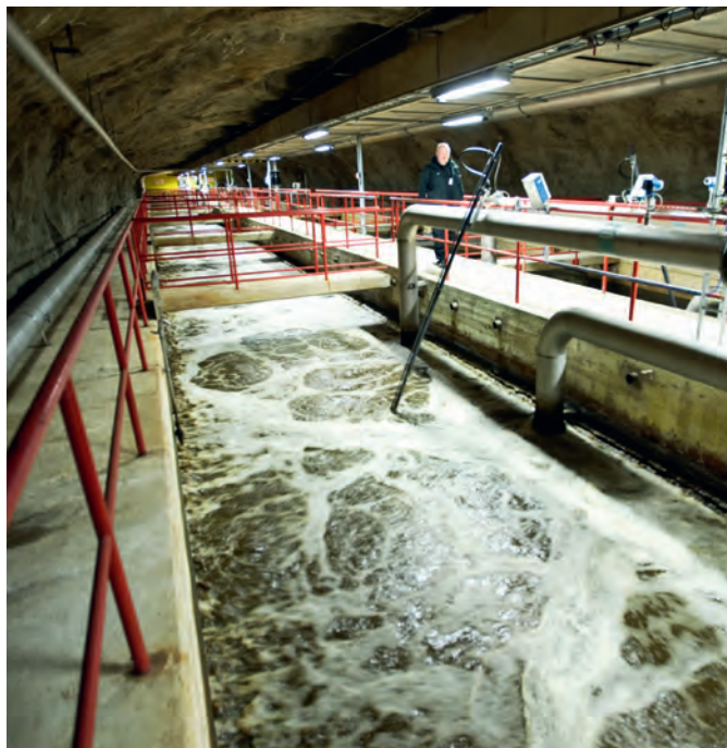
Aeration basins for biological treatment of wastewater with the activated sludge process. Left: basin in operation. Right: basin emptied for inspection. Photos: ©Kari Kohvakka, Stockholm Vatten och Avfall.
