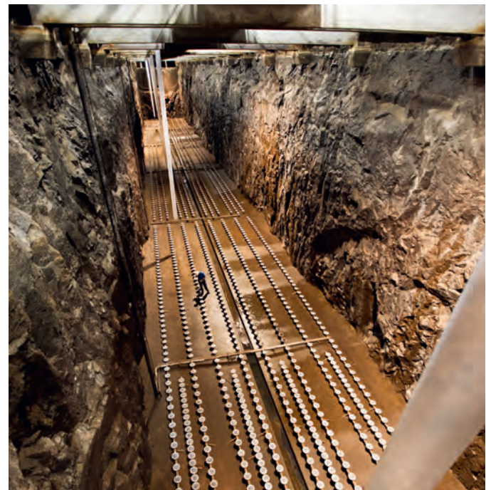
Aeration basins for biological treatment of wastewater with the activated sludge process. Left: basin in operation. Right: basin emptied for inspection. Photos: ©Kari Kohvakka, Stockholm Vatten och Avfall.
