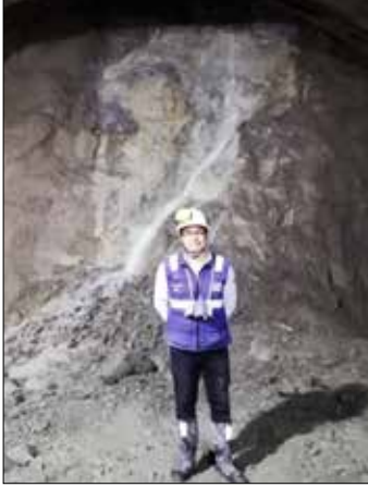
Juan Pablo Romero at his day job on the Tesalia Tunnel
