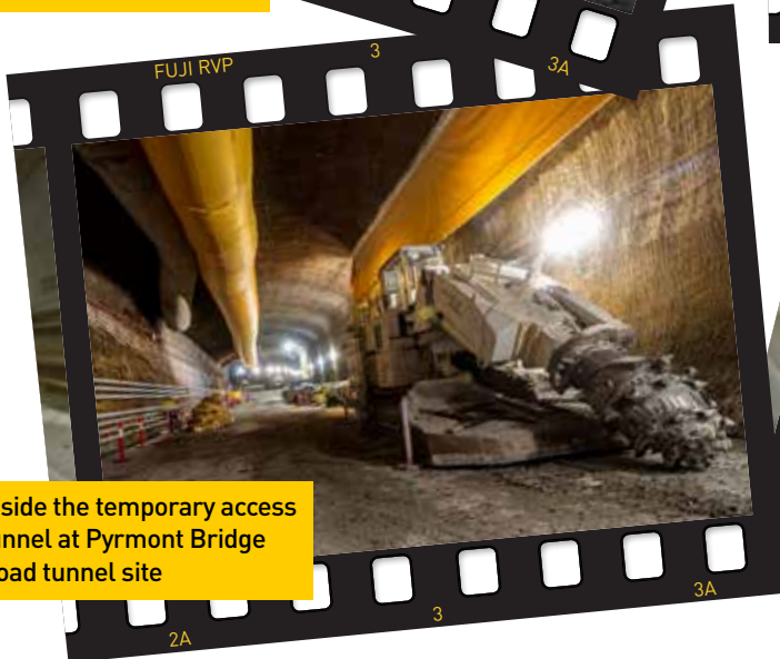
A 135 tonne roadheader excavates sandstone
